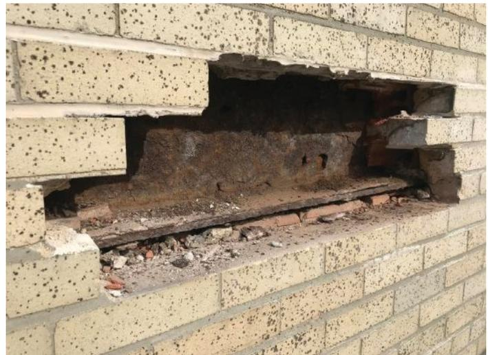
*Test cuts can provide insight into the existing layers, securement methods, and material conditions.*
