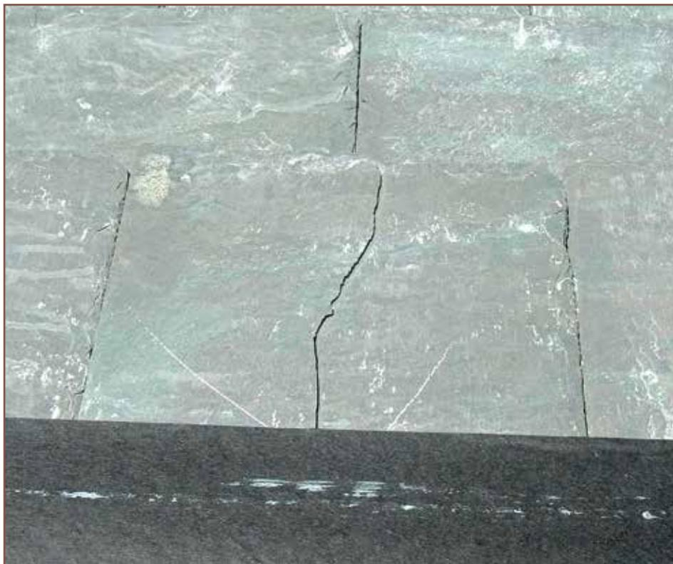
Figure 5 – Cracked slate.
