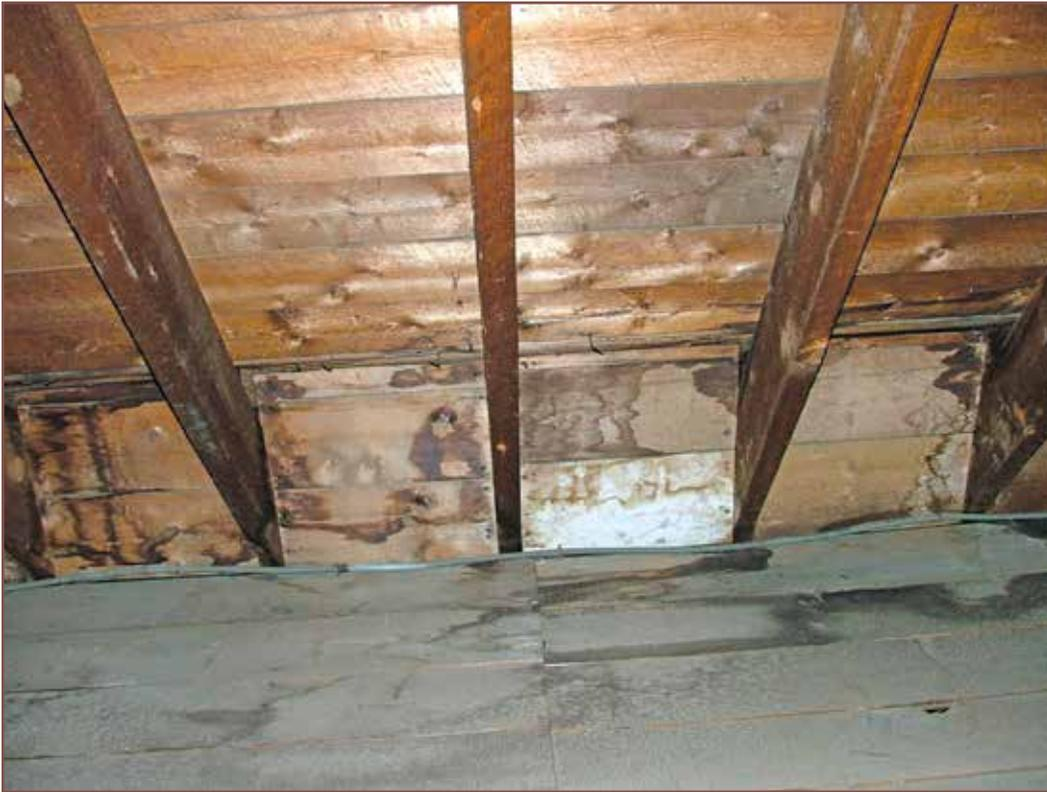
Figure 4 – Staining under roof deck and on floor.
