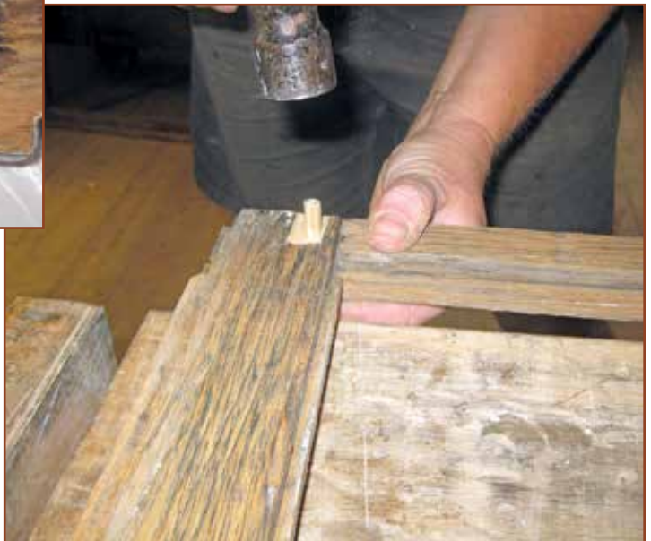
Photo 4 –Dutchman repair of wood sash corner.
