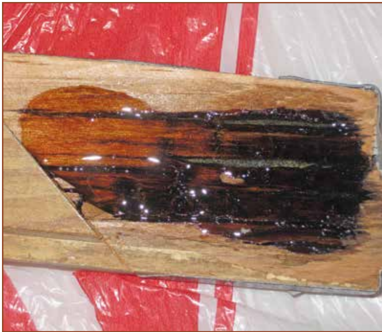
Photo 3 – Epoxy repair of checked wood with resin.
